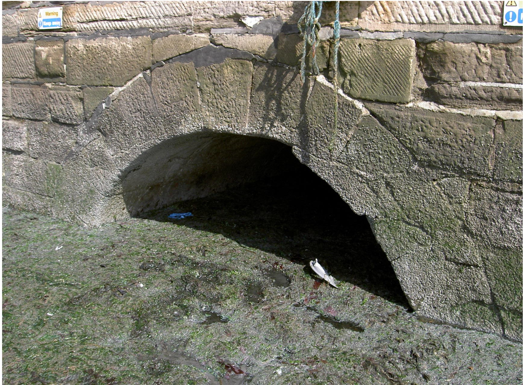
Margate Harbour Sluice –open end of culvert viewed from inner face of Stone Pier
